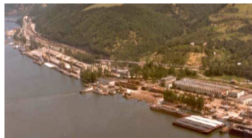
Figure 4. Port Orșova, commercial area.
