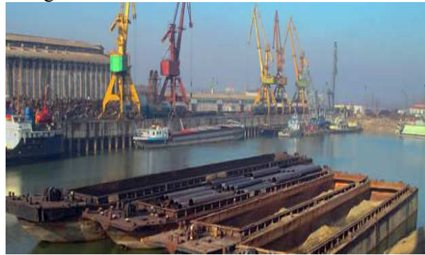
Figure 12. Braila Harbor, commercial area. Source: "Hercules" SpA Company Brăila.
